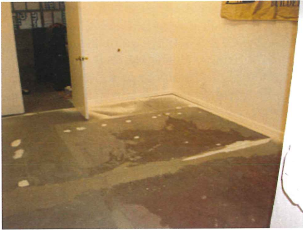
The work to make the 2005 expansion of space usable has been hard. Trustee Mark Brown had to strip the floor in a large room, and then lay down epoxy paint.
